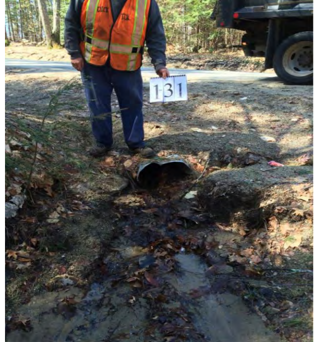
PHOTO of town culvert ~ assessed & prioritized for replacement
