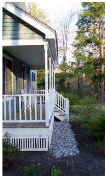
Another example of a drip edge along roofline.
