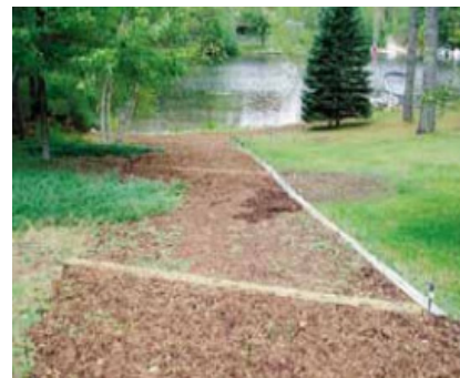
Waterbars along the path slow flow and divert runoff into vegetated areas.
