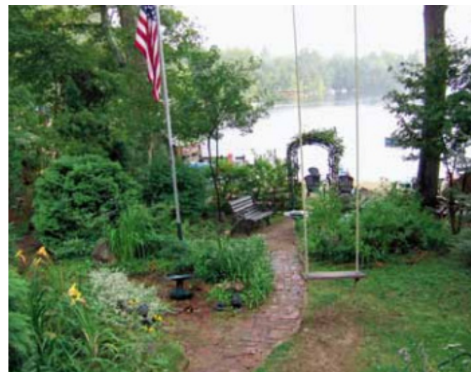
PATHWAYS made of semi-permeable pavers meanders to water. Runoff is distributed into vegetated gardens where it infiltrates the ground before reaching the shore.
