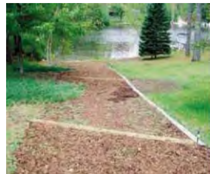
Waterbars along the path slow flow and divert runoff into vegetated areas.
