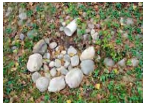
A plunge pool is an area where water is collected and allowed to infiltrate.
