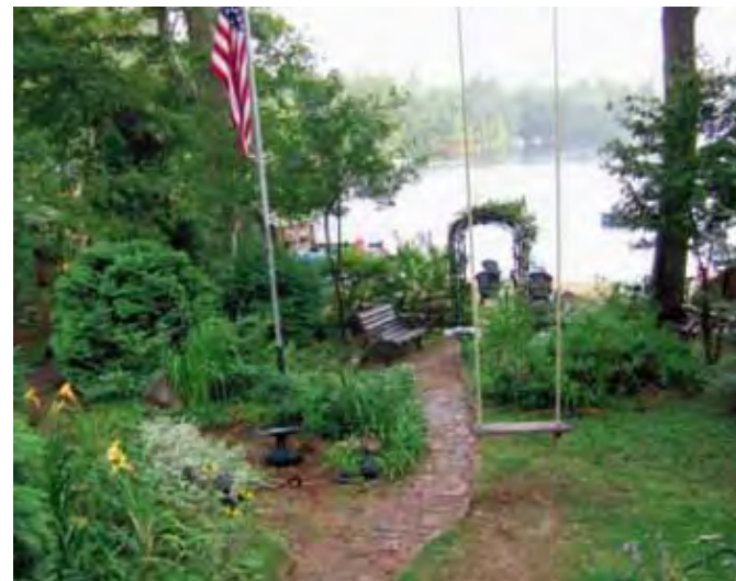
PATHWAYS made of semi-pervious pavers meanders to water. Runoff is distributed into vegetated gardens where it infiltrates the ground before reaching the shore.
