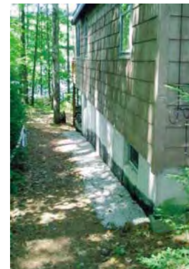
An infiltration trench was constructed to catch roof runoff at this lakeside home.
