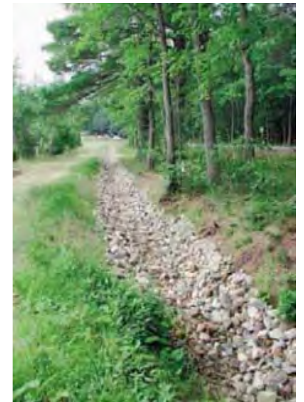
A swale constructed along this roadway captures road runoff and prevents it from entering the lake, to the left.
